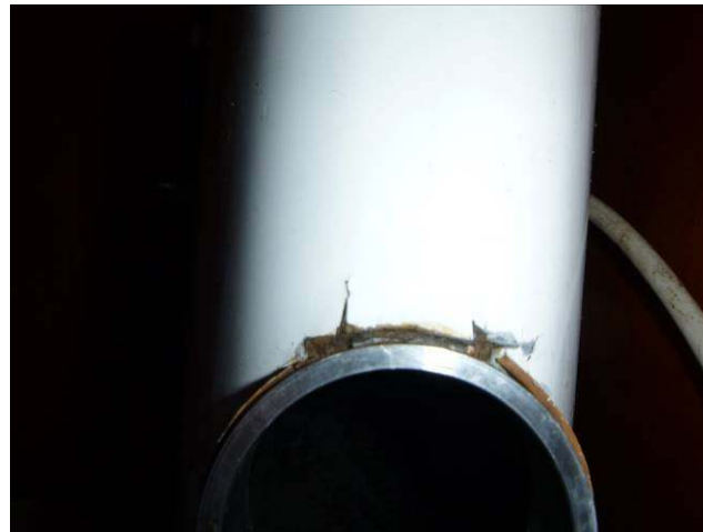
Mast, perimeter of sleeve for mast jacking pin near base
