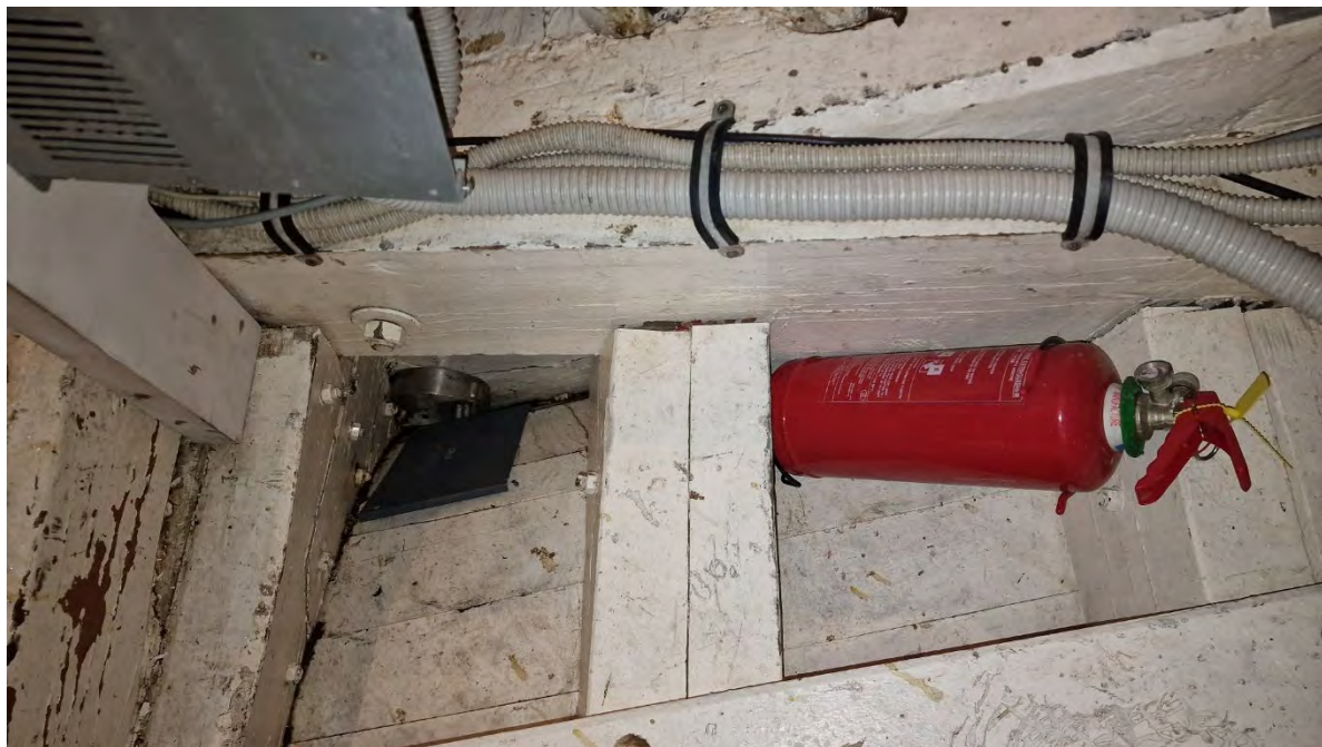
Photo 53 Engine room bilge area.
