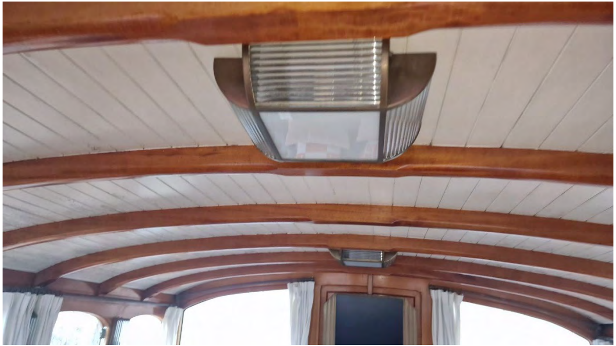
Photo 27 View of ceiling in way of saloon area.
