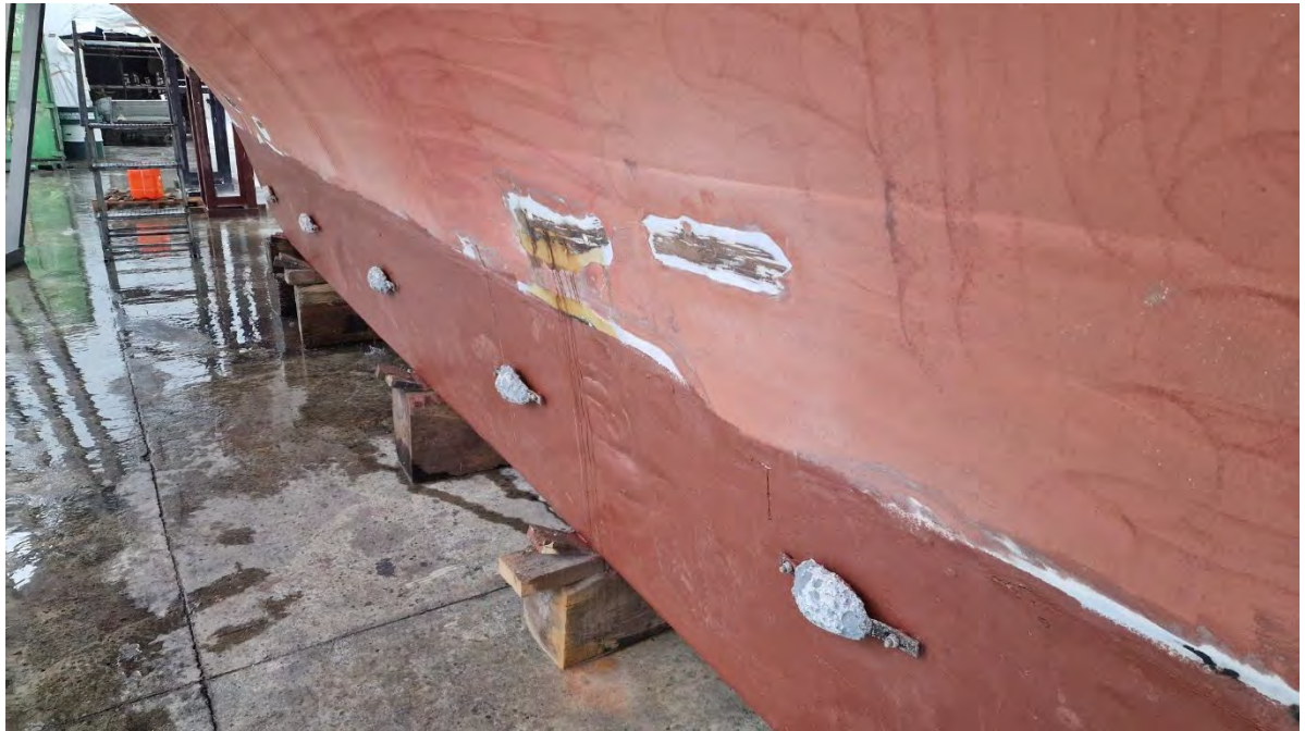
Photo 25 Spot maintenance works in way of the port side underwater hull area.
