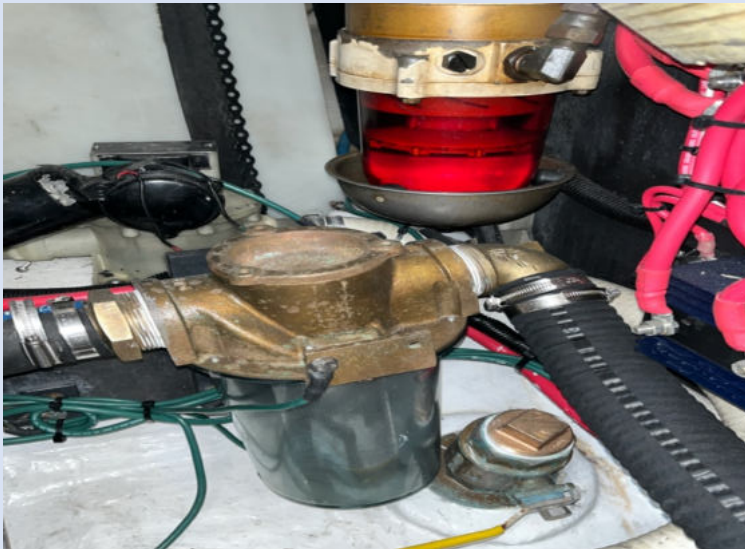
Rubber raw-water hoses, thru-hulls, seacocks, valves, sea-strainers, grounding wires, Racor diesel fuel-water separating filters & Fireboy suppression system is new
