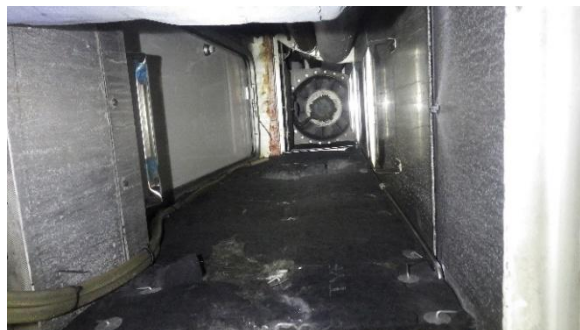
MAIN ENGINE ROOM EXHAUST FANS INSTALLED WITHOUT PROTECTIVE GUARD/SCREENS
