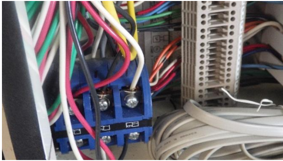
PINS OR FERRULES ARE NOT INSTALLED ON WIRING WITHIN HVAC ENCLOSURE COLOR CODING IS TO NO RECOGNIZED STANDARD. RAW WATER SWITCH NOT LABELED
