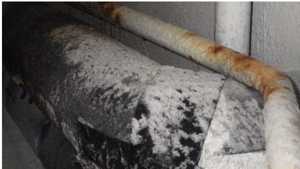
NO AIR INTAKE SCREEN ON MISC. FCU'S
