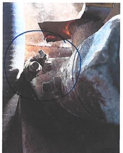
BROKEN BONDING WIRE
