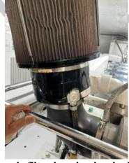
We can see in the photo the air filter housing has had a modification. Filter was working but recommend cleaning or replacement.
