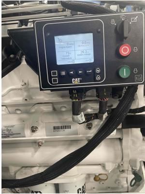
● 2.5 Inspect Engine Wiring & Harness
