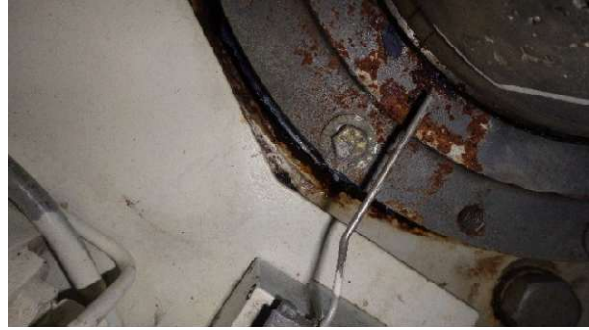
WATER LEAKING FROM PORT FIN
