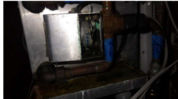
WIRE JOINTS AND MOLDY WATER VALVES THROUGHOUT FAN COIL
