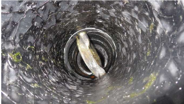
PORT ABOVE WATER M/E EXHAUST
