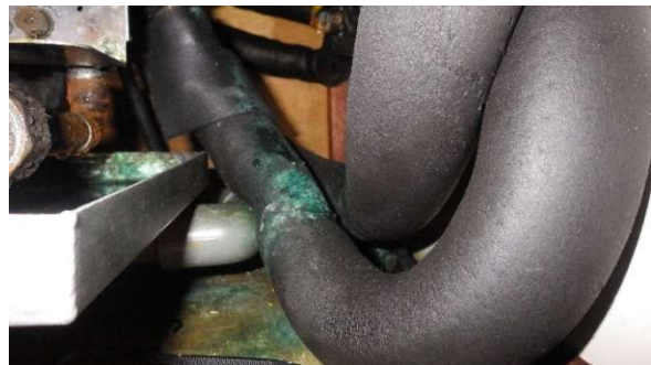
MOLD OBSERVED THROUGHOUT THE YACHT WITHIN MULTIPLE FAN COIL UNITS
