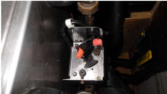
WIRE JOINTS AND MOLDY WATER VALVES THROUGHOUT FAN COIL
