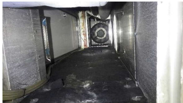
MAIN ENGINE ROOM EXHAUST FANS INSTALLED WITHOUT PROTECTIVE GUARD/SCREENS
