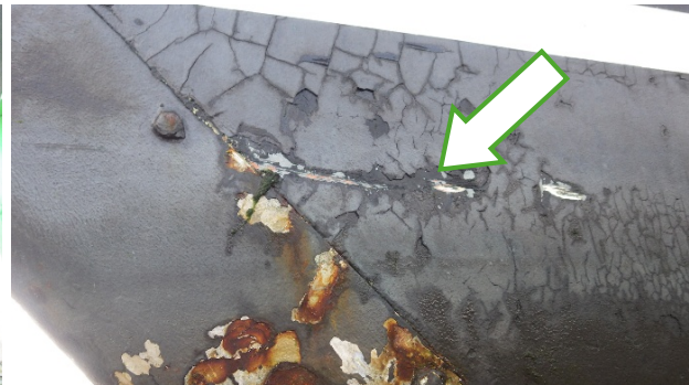
DISBONDMENT NEAR THE BOTTOM PAINT STAINLESS CUT WATER AT THE BOW. HEAVY PAINT AND GOUGE OBSERVED
