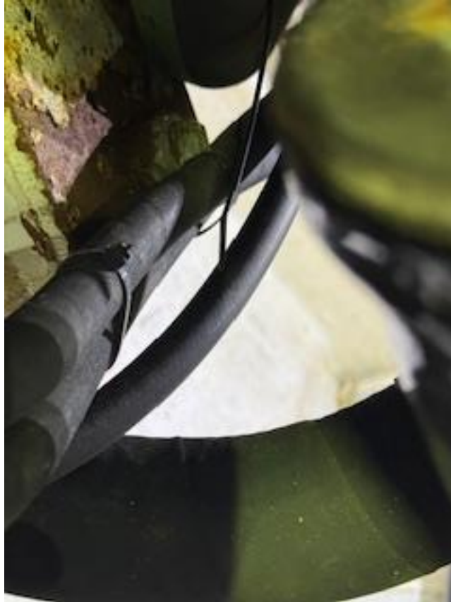
The starboard transmission cooler hoses are chaffing on the right rea engine mount.
