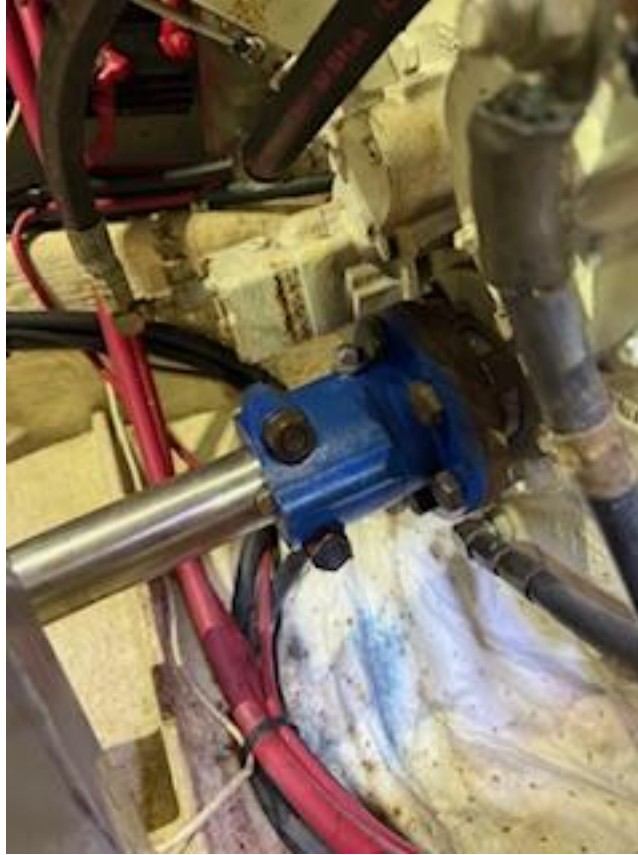
The port prop shaft appears to have been recently replaced.
