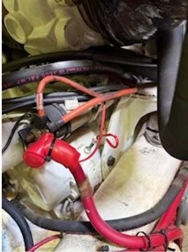
Port engine starter wiring is chaffing on the right rear engine mount.
