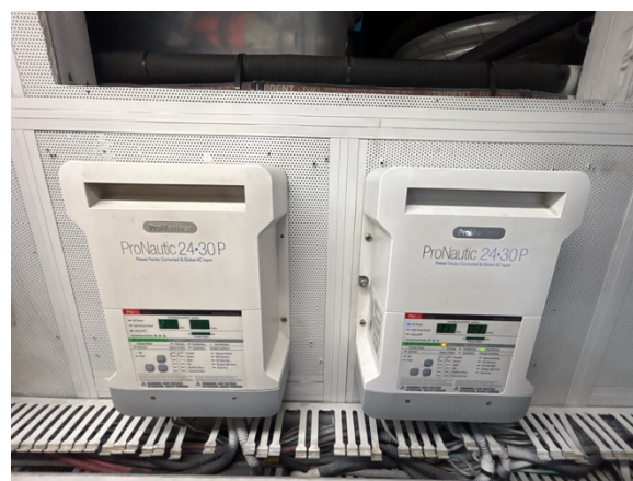
Engine and generator battery chargers
