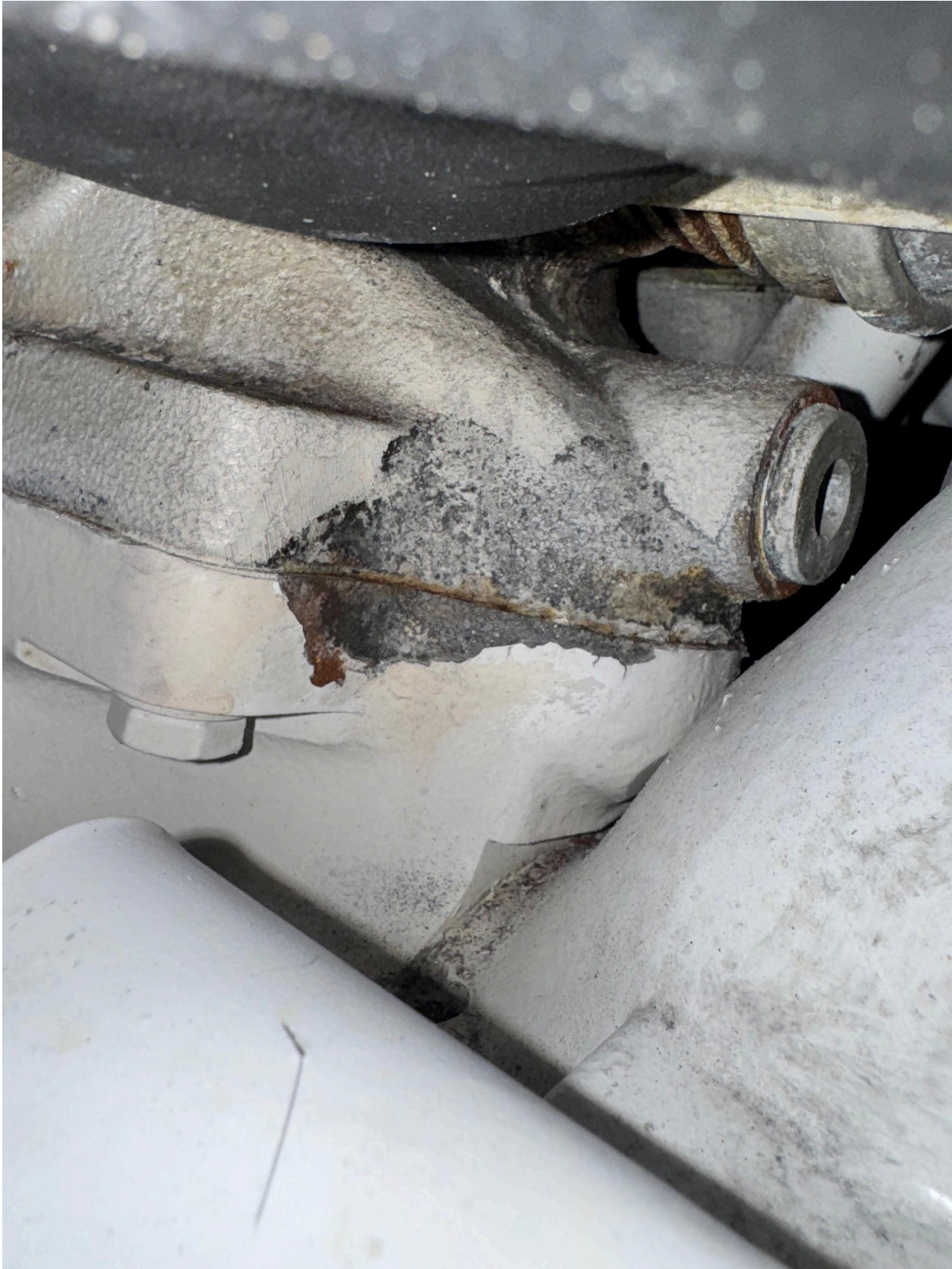
STARBOARD BOTH TURBOS CORROSION AND START OF COOLANT LEAK
