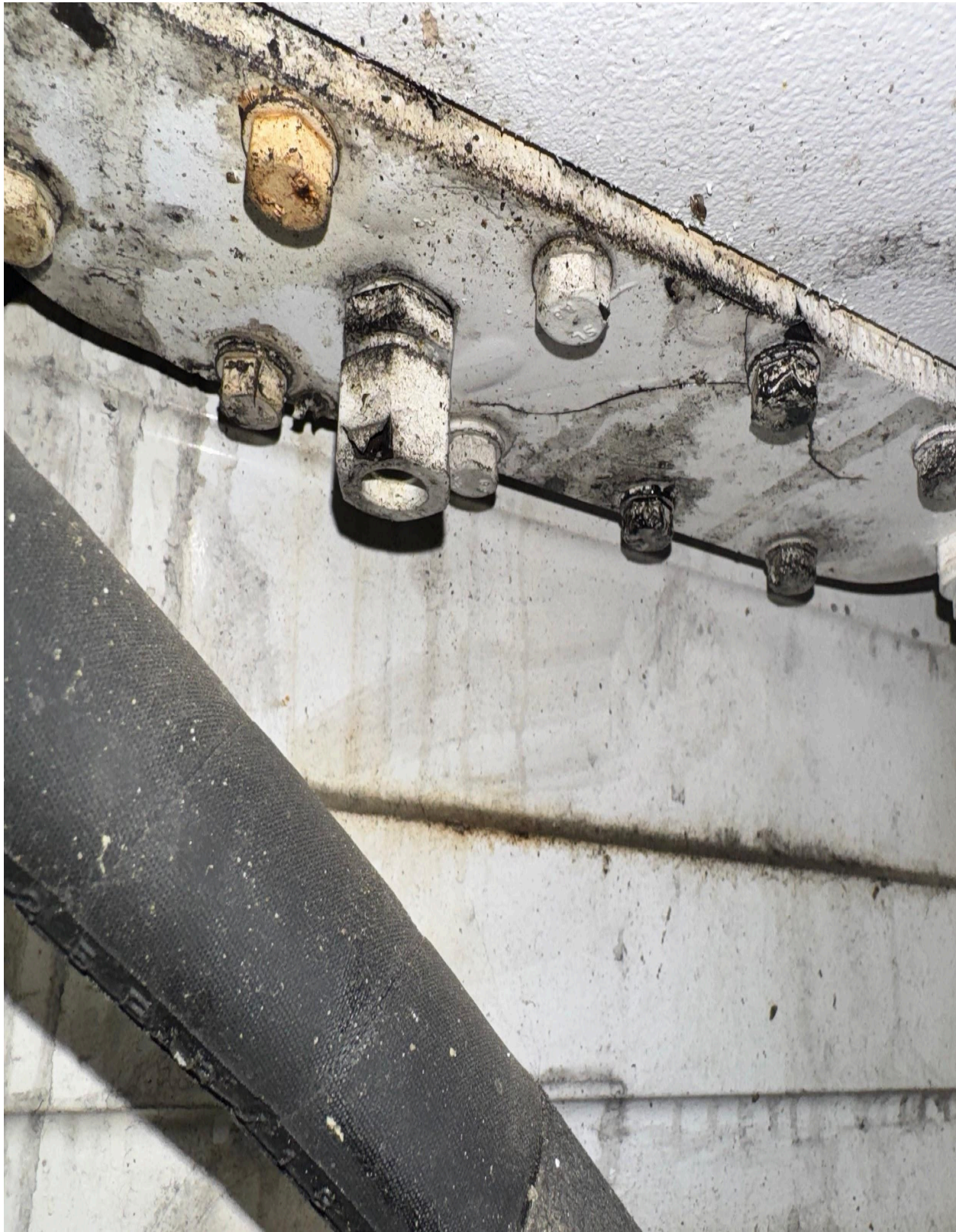
STARBOARD FLY WHEEL COVER SEEPING OIL
