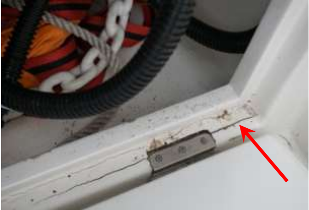
Figure 10.25 Crack/split in cockpit storage locker
