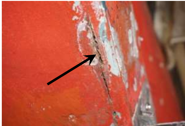
Figure 10.14 Flaw at lifting-rail hull interface
