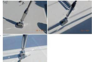
**Ends:** Secure and no split or corroded ends/wires.
