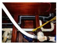
**Supply lines:** Grey plastic piping and PVC water lines. No leaks sighted.
