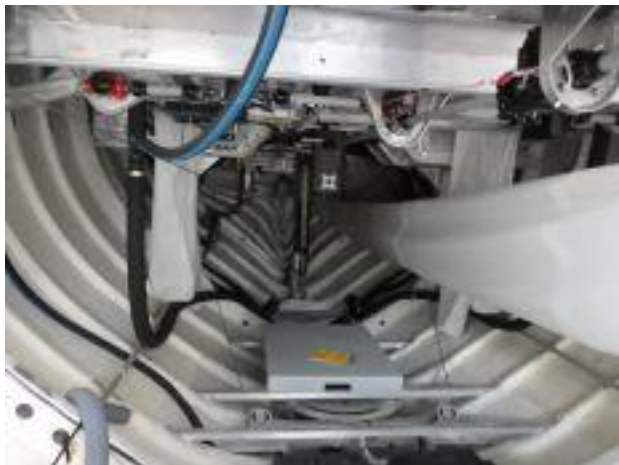
Looking aft from trim tab quadrant
