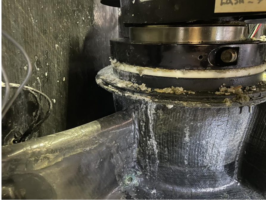
Above shows the leaking at the rudder bearing
