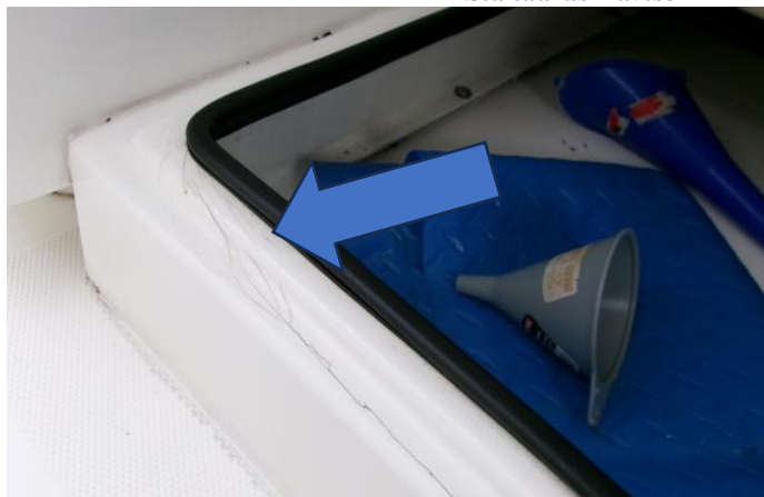
Stress Cracks on the hull
